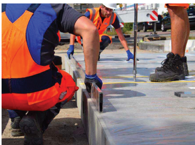
Fig. 11: Levelling by implemented adjustment system
