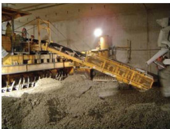
Figure 5: Two layer concrete pavement, wet-in-wet: supply of concrete of the upper layer over the first slipform paver
