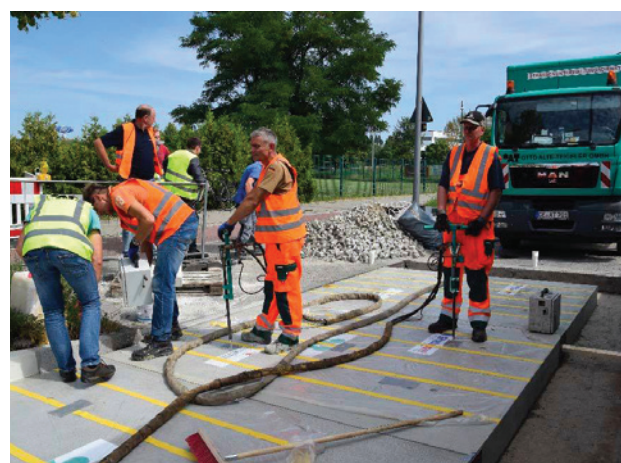
Fig. 12: Injection of the silicate resin to fill the hollows
