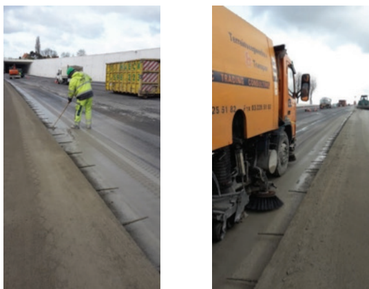
Figure 12: Cleaning of the asphalt layer next to freshly placed concrete after exposure of the aggregates at the surface
