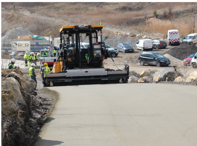
Picture 3: Paving process
