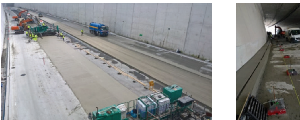
Figure 7: Construction of the two-layered concrete in the open trench and tunnel
