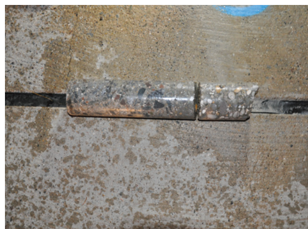
Fig. 6: Drill core of a concrete slab and bearing course without bond
