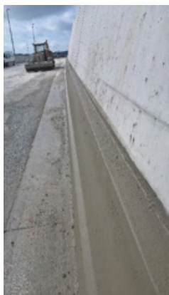
Figure 11: Exposure of the aggregates at the surface of the CRCP
