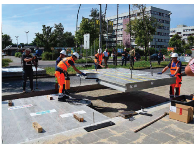
Fig. 9: Laying by stud bolts
