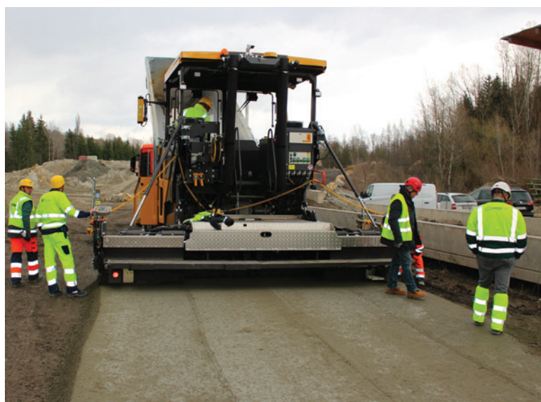
Picture 2: Paver with the high-compaction pile
