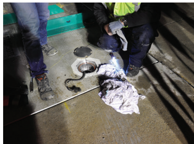
Fig. 8: Pulling the cable of the light signal
