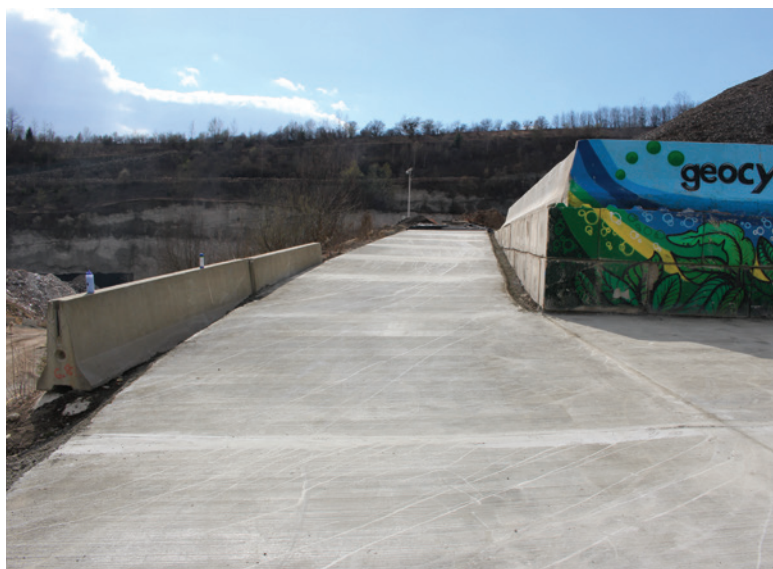
Picture 5: Realized surface after cutting the joints
