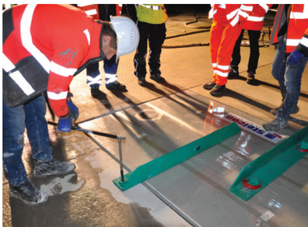
Fig. 7: Levelling of the slab by traverses through the cable slot
