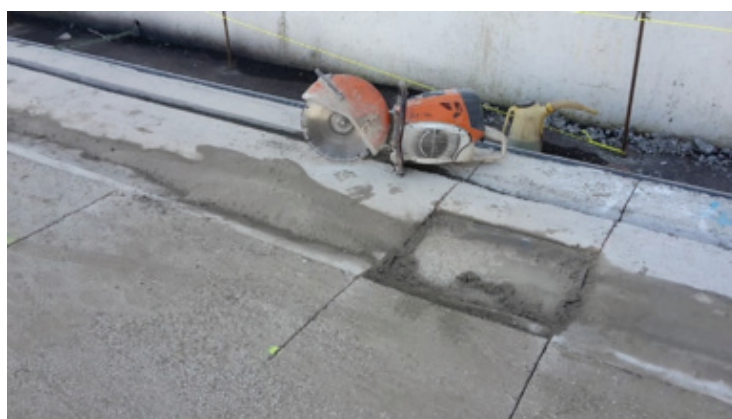
Figure 6: Cutting of the active crack control immediately after washing of the surface each 1,20m. At the height of the gully (still covered with plastic), an extra saw cut is applied
