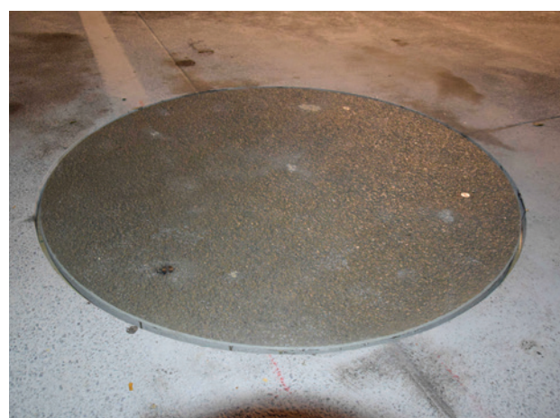
Fig. 4: Installed round precast slab
