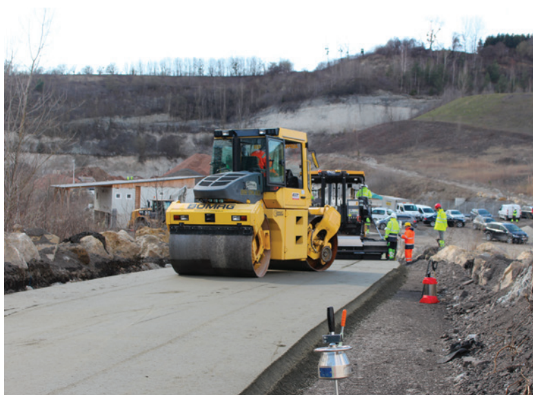
Picture 4: Compaction with drum roller
