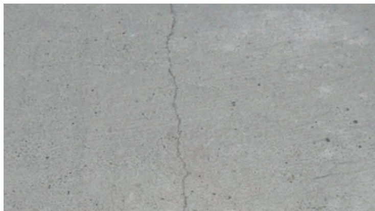
Figure 11: Exposure of the aggregates at the surface of the CRCP
