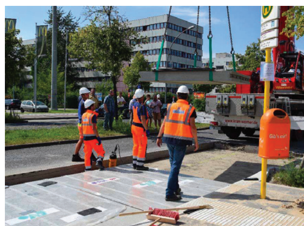
Fig. 10: Laying by belts
