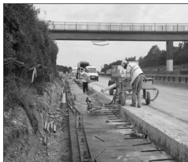
Install tie bars
