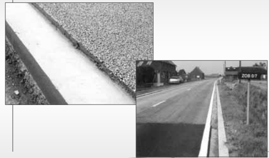
Herne, 1996 - test sections of low noise surfaces
