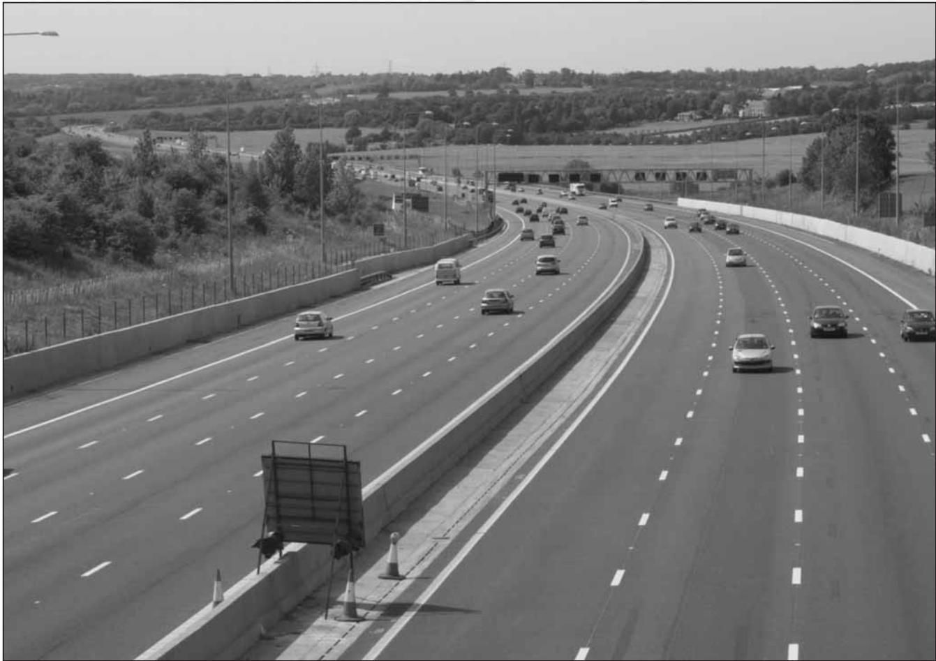
A section of completed Dual 4 lane motorway incorporating most of the slip formed concrete components used on the M25 project.
