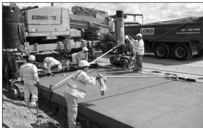
Gomaco paver laying new Pavement Quality hard shoulder
