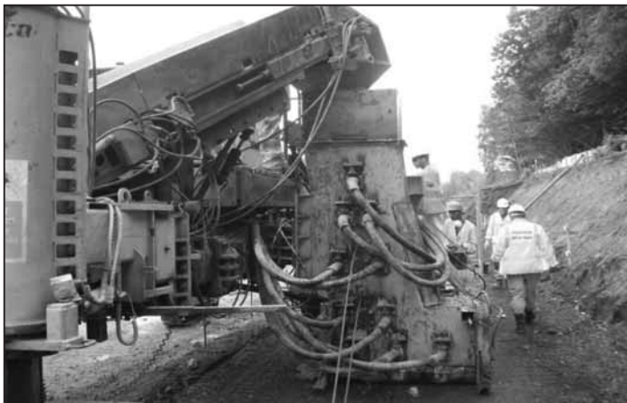
A complex mould was required to produce the 'L' shaped section
