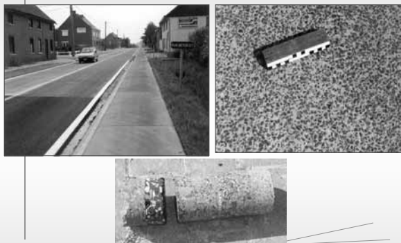
Herne, 1996 - test sections of low noise surfaces
