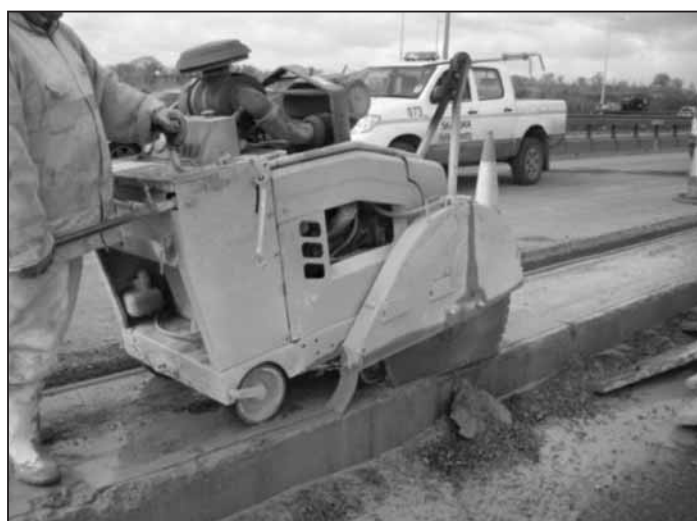
Saw cut pavement edge
