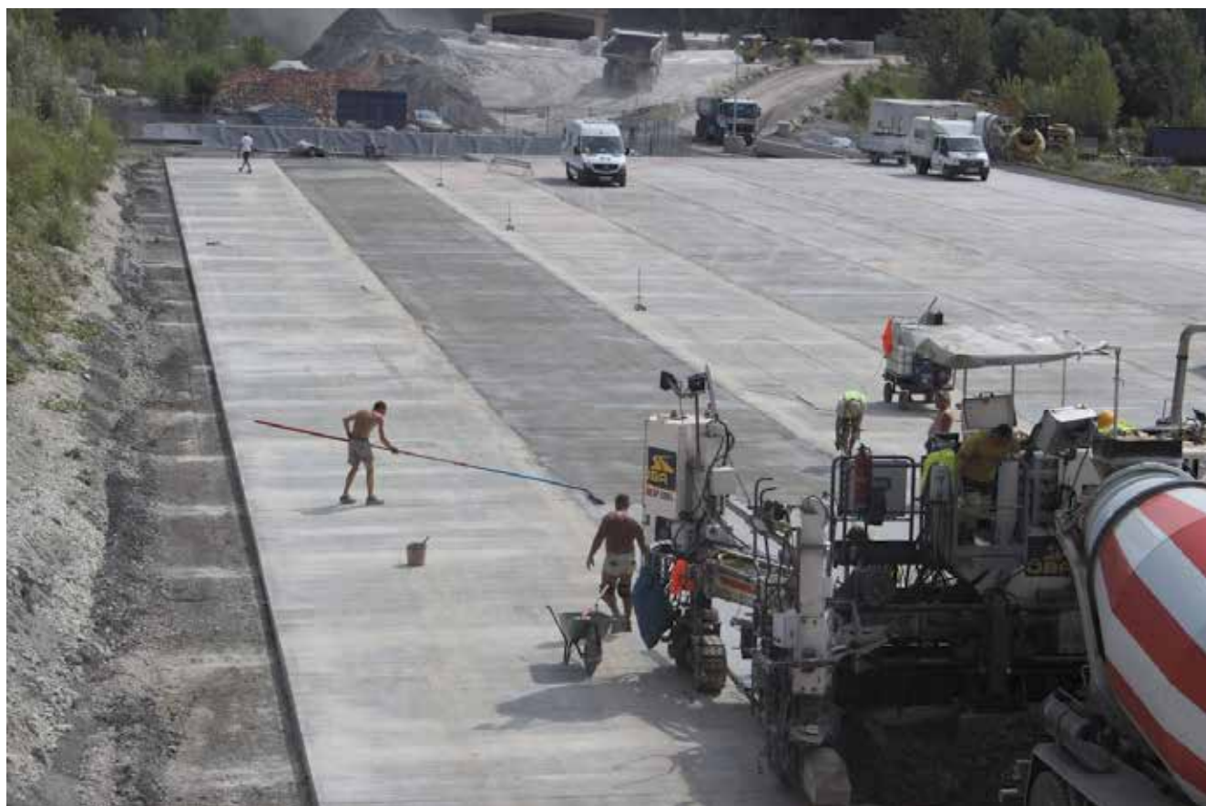
Picture 1) Concrete paving of the testing area
