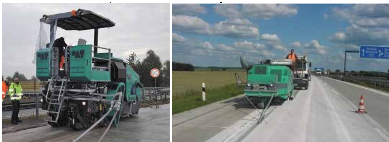
Picture 4) Diamond grinding in Germany
