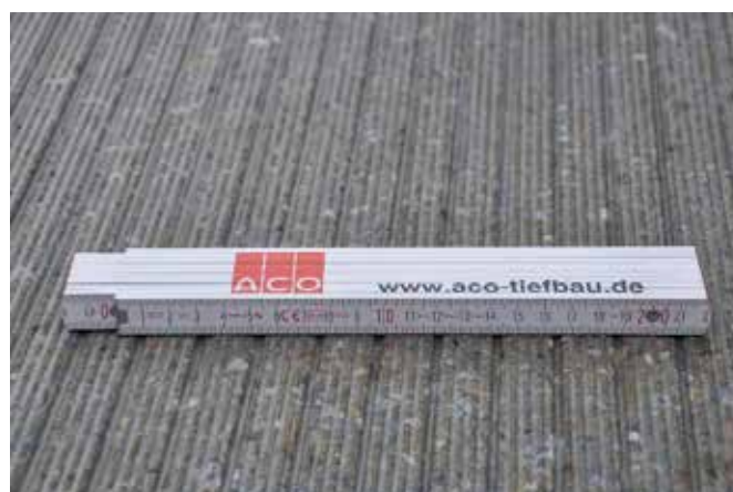
Picture 6) grinding and grooving, distance of grooves 20mm (source VKI)
